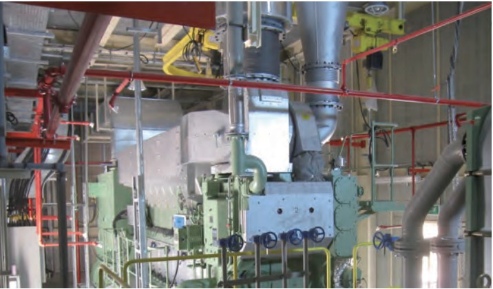
Inside view of Enclosure(Pre-fabricated type)
